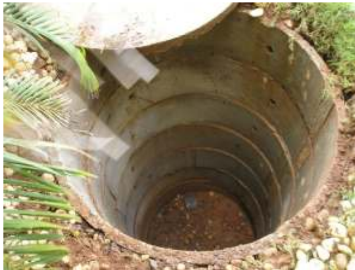
A recharge well
