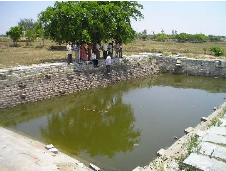
A traditional 'kalyani' to store rainwater
